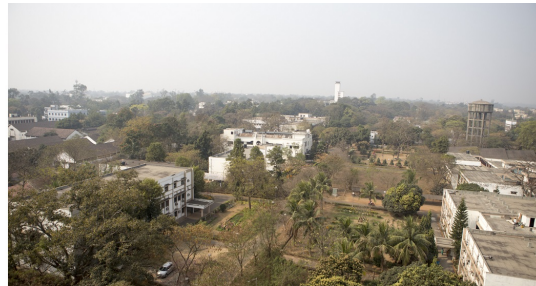
Figure 3.1: Exterior view of the CORAL Institute ( left ), View from the roof of the building ( right )
